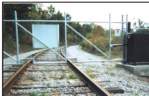
Custom Curb Notch
